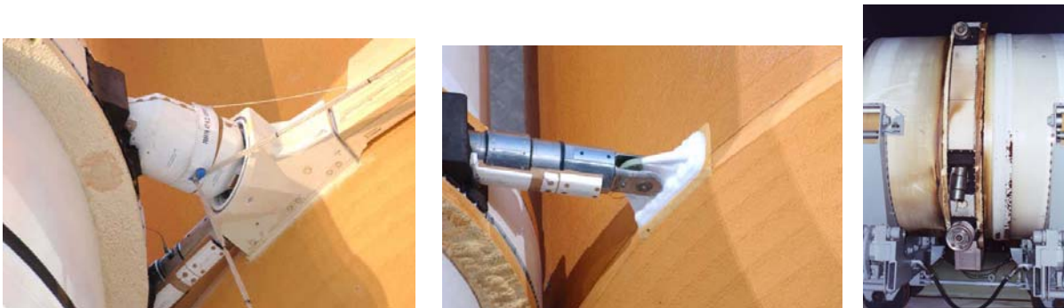
Figure 3-14. External Tank Attach Ring Showing Pre and Post Separation Strut Condition.
